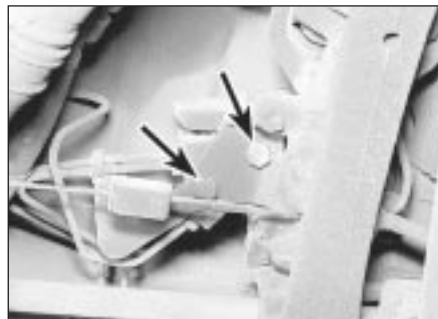
21.4 Rear brake pressure-regulating valve securing bolts (arrowed)
